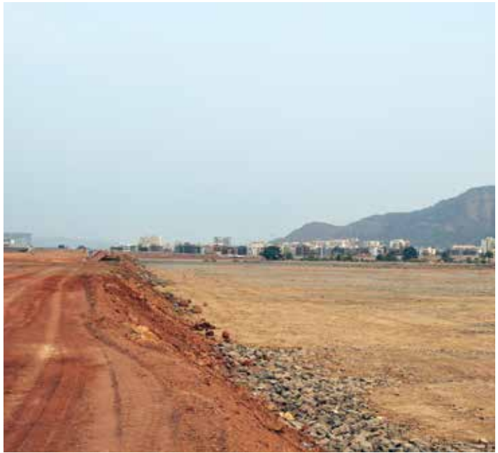
Land-filling and construction in the proposed NMIA area
